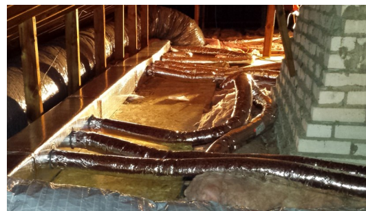
Unico System Square supply plenum
