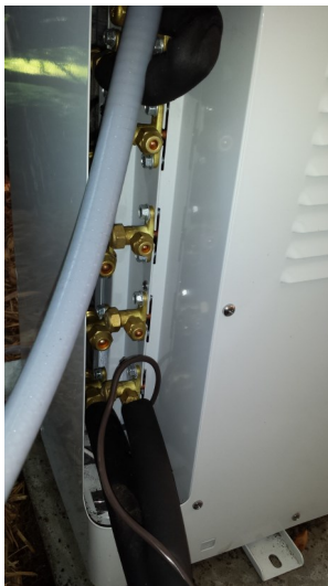
Flare connections make installation a breeze
