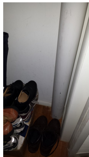
This small pipe located in the closet was all that was needed to run duct in between floors
