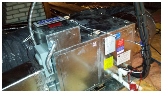
Unico iSeries blower and coil installed in attic
